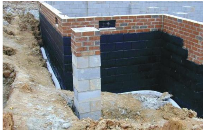
The below-grade concrete walls have damp-proof coating
