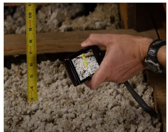
Figure 1. Measuring the depth of attic insulation.
